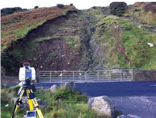
Figure 2: Leica HDS3000 Scan station, Terrestrial LiDAR scanning surveying slope morphology, Co. Antrim, Northern Ireland.
